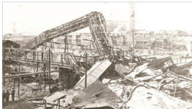
Aftermath of the Chilwell Explosion
